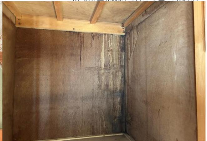
2階6帖和室(南側)押入壁の雨漏り痕
